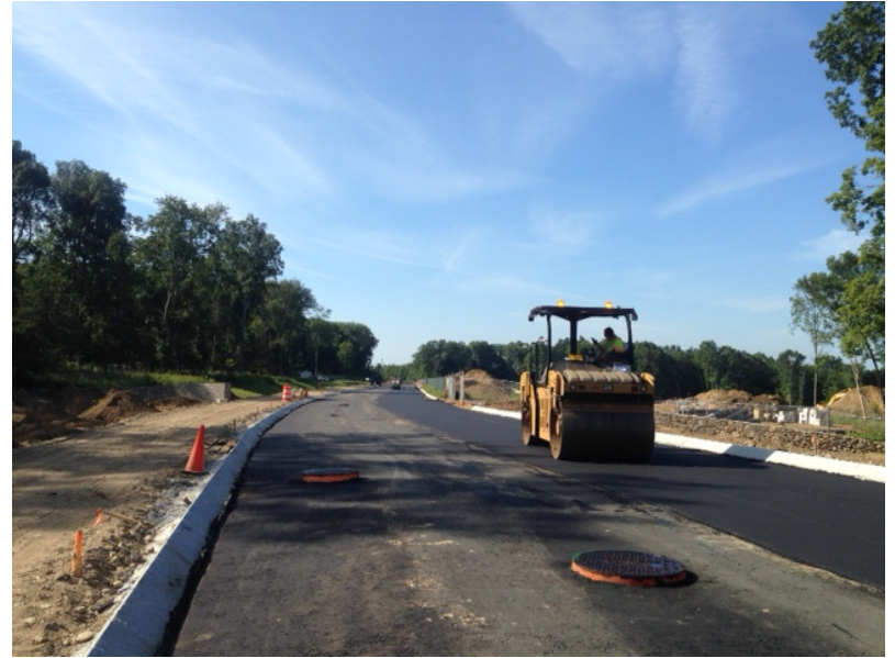
Base Course Paving in Progress
