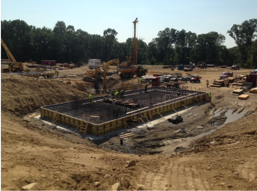
North Lab Bar Support Tower Foundation Reinforcement
