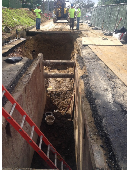
Sewer replacement – Storrs Road in front of Blake House Trenching and Rock Removal
