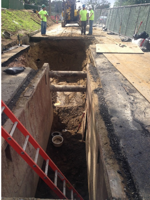
Sewer replacement – Storrs Road in front of Blake House Trenching and Rock Removal
