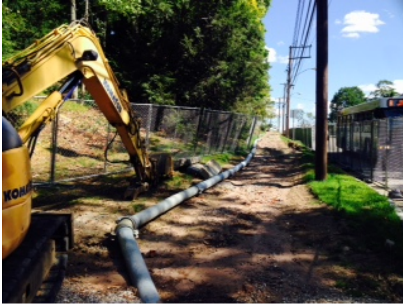
Sewer By-Pass Piping and Pumps – Storrs Road – to allow for sewer replacement
