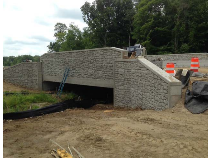
Box Culvert Construction at Wetlands Crossing A
