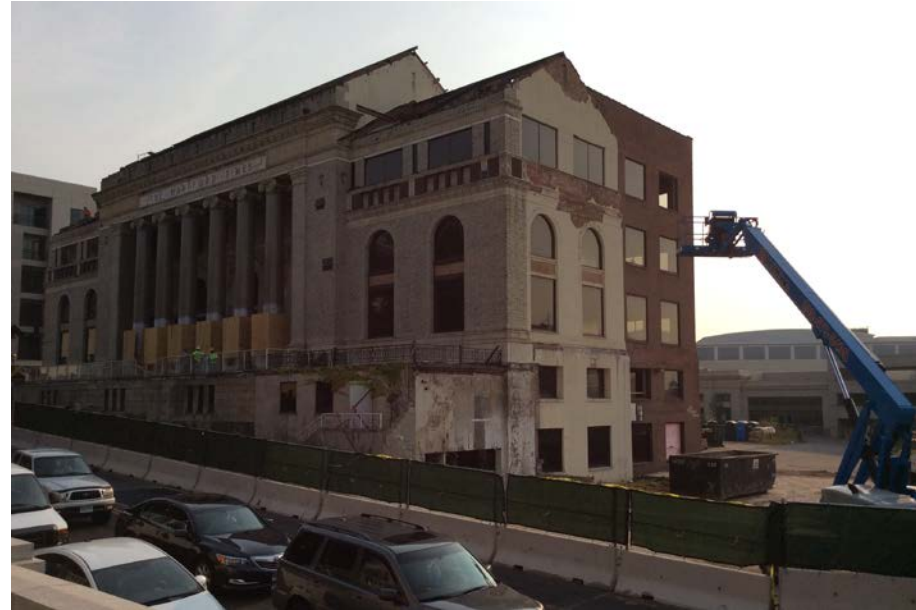
Construction on the Hartford Times Building
