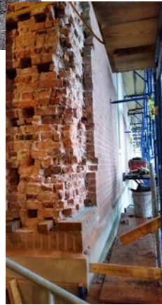
Masonry Repairs, right
