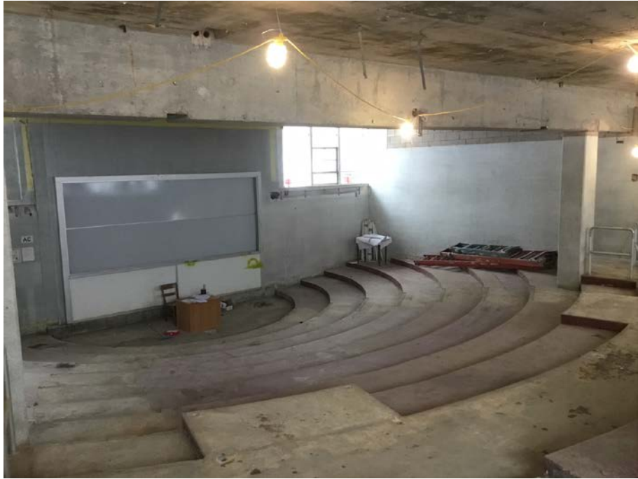
Monteith Lecture Hall
