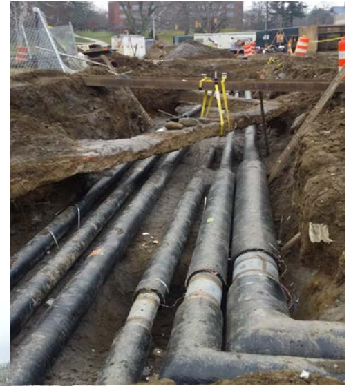
New Steam & Condensate Return Piping
