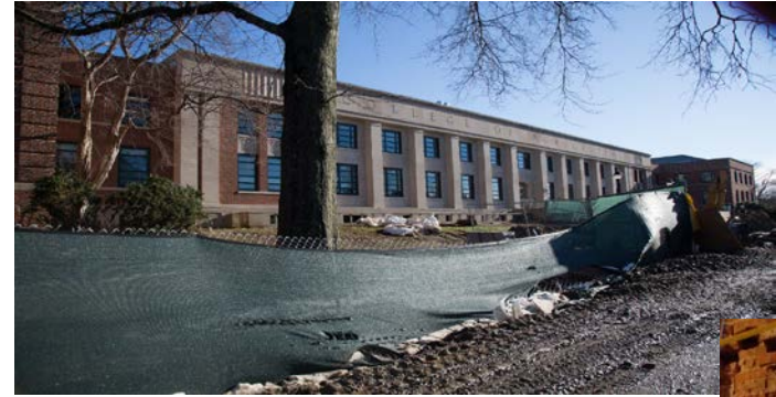
West façade of Young Building, top
