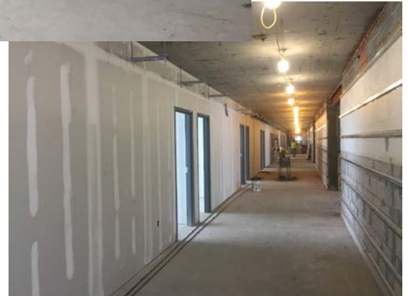
3 rd floor classrooms, above 2 nd floor corridor, below
