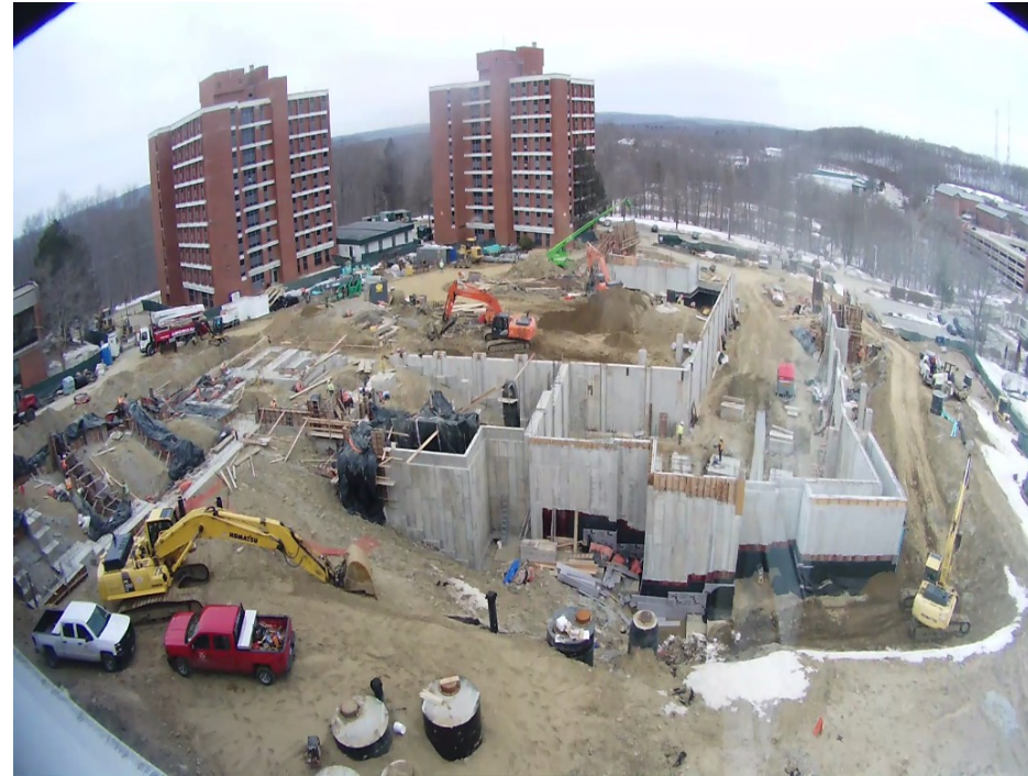
View looking North
