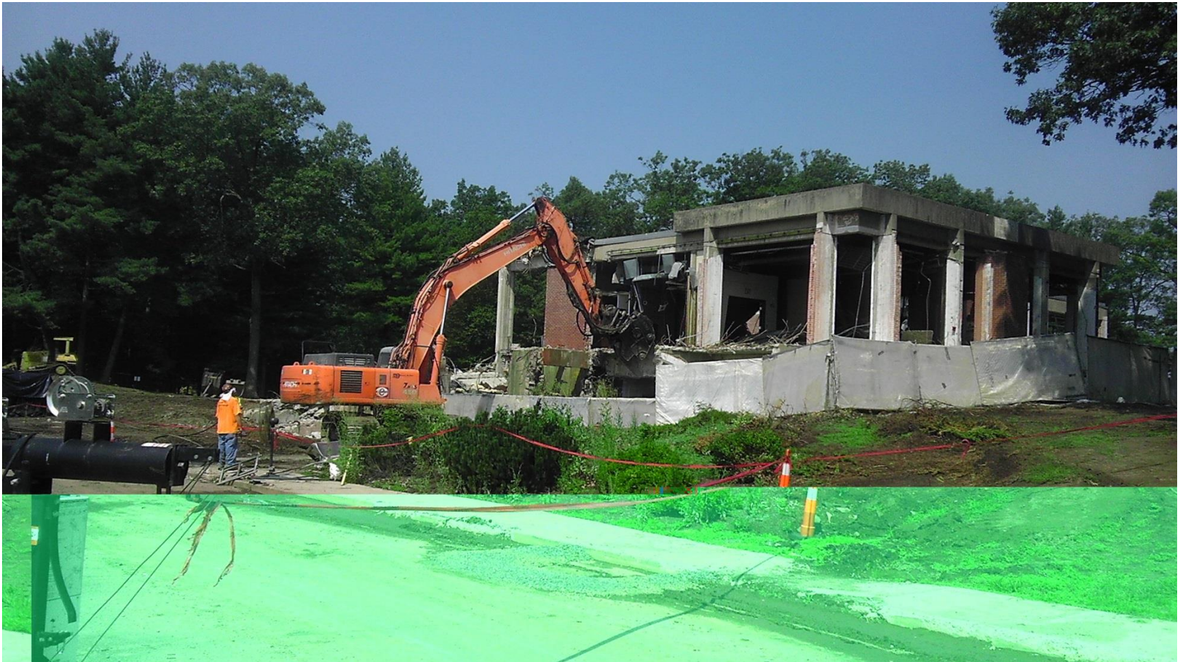
Detail of Hitachi 450 Hydraulic excavator with a pulverizer attachment
