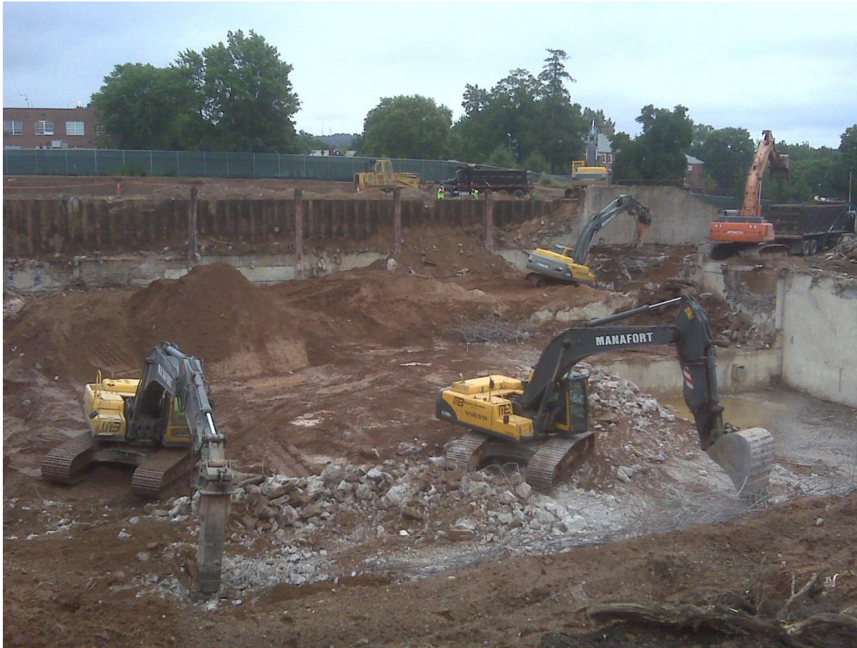
Detail of several hydraulic excavators (Volvo EC-290 and Volvo EC-360) with a hydraulic Hammer and bucket attachments
